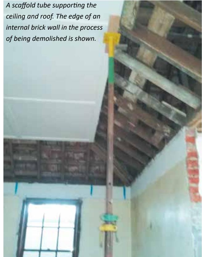
*A scaffold tube supporting the ceiling and roof. The edge of an internal brick wall in the process of being demolished is shown.*
