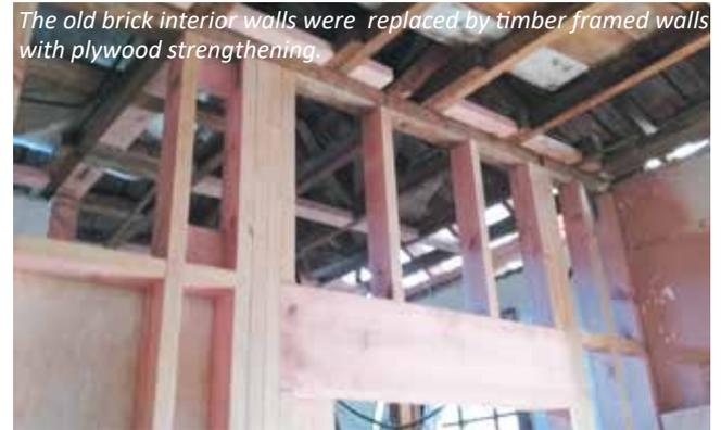
*The old brick interior walls were replaced by timber framed walls with plywood strengthening.*
