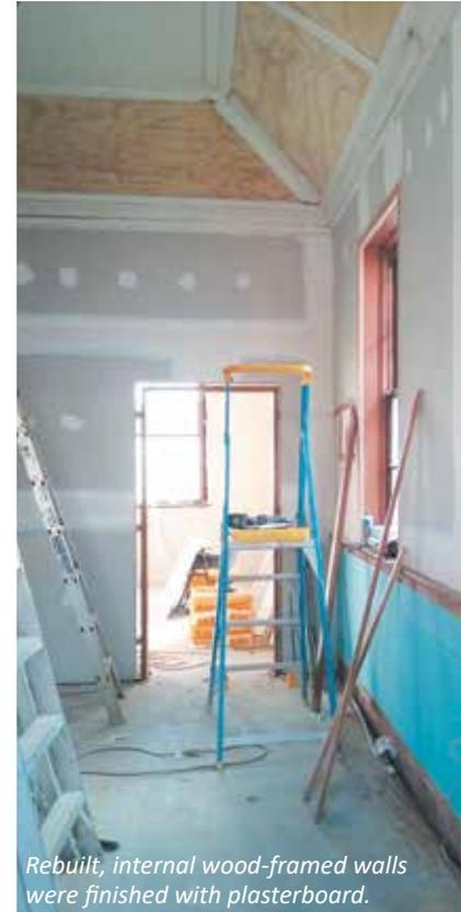
*Rebuilt, internal wood-framed walls were finished with plasterboard.*
