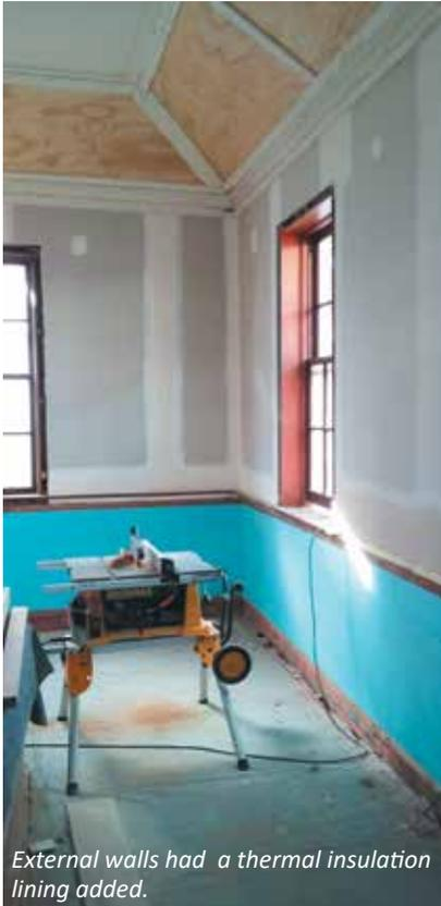
*External walls had a thermal insulation lining added.*
