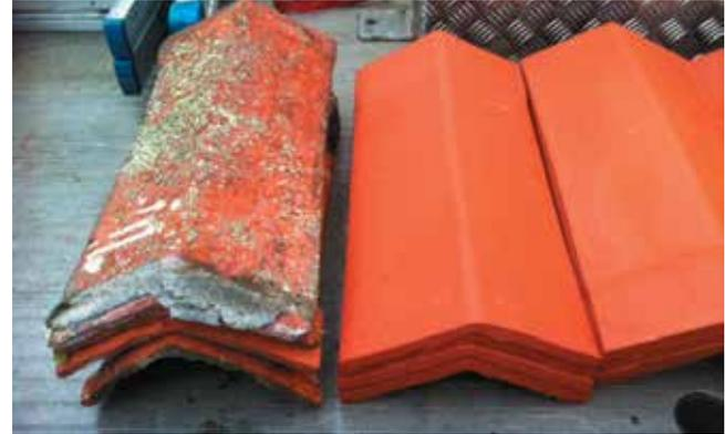
*Ridge tiles were cleaned and broken tiles replaced.*
