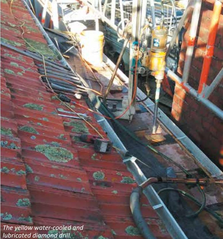
*The yellow water-cooled and lubricated diamond drill.*
